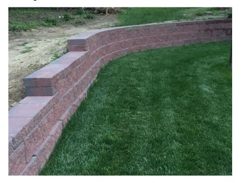
Sod and a retaining wall have been added behind the fence. This is great news for the league. Rushing water and rivets of dirt have been an issue in past seasons. The retaining wall will prevent water from doing any damage to the field throughout the year and it gives teams a great place to sit. Yay!
